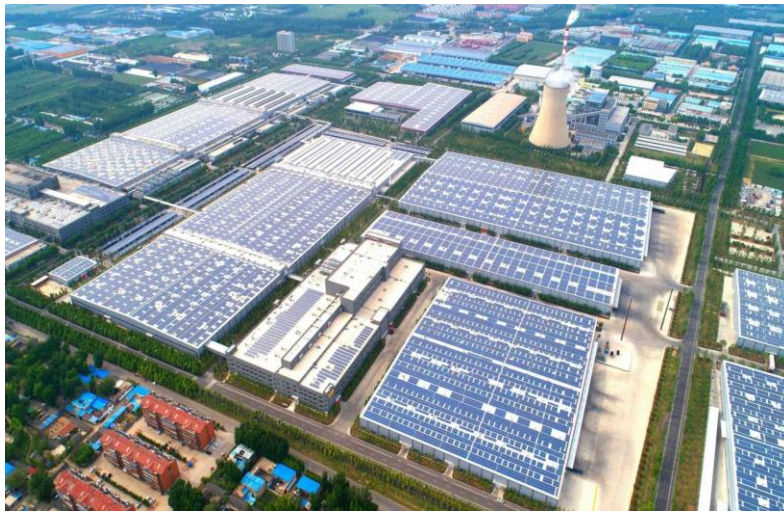
Figure 13: World's largest C&I installation, Jining, Shandong, China (Source: Hill, 2021)
