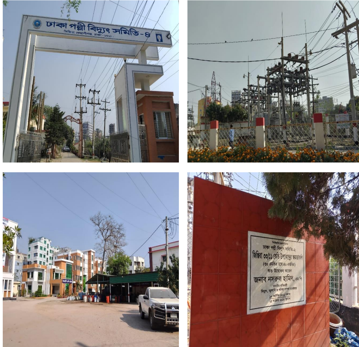
Figure 7-5: Substation Situated 2.5 km from Proposed Site
