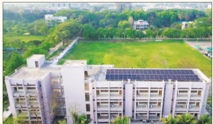
Net Metered Rooftop Solar System at Khulna University
