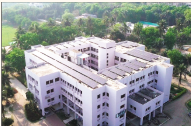
Net Metered Rooftop Solar System at Khulna University
