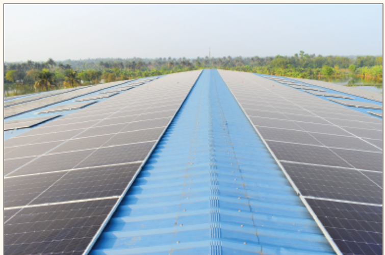
Net Metered Rooftop Solar System at HMCL Niloy Bangladesh Ltd.
